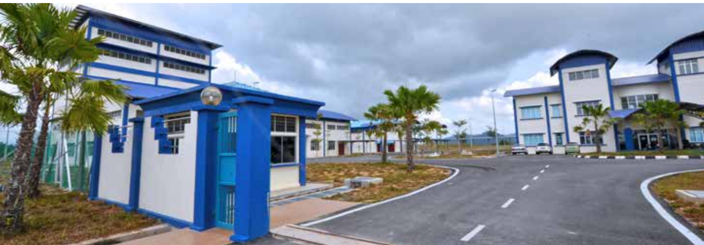
Bangunan Loji Rawatan Air Panching
